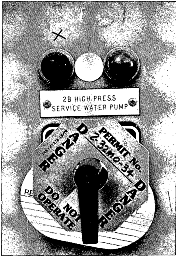
Figure 4.17 Placement of a Blocking Tag in BWR Control Room (Caution Tag is Visible beneath Blocking Tag)
